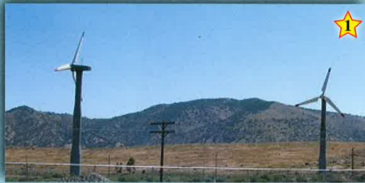
Danish turbines circa 1984 65 kw 15 meter or 50 foot towers
